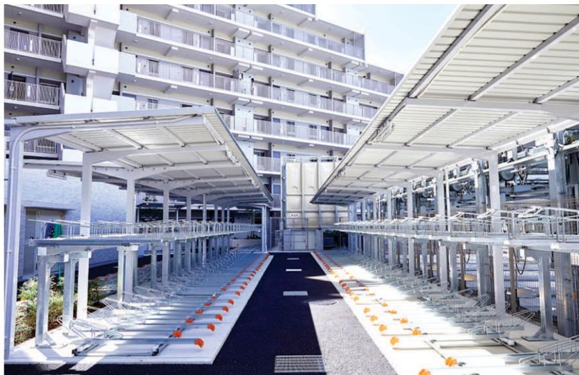
Bicycle-parking lot at The Parkhouse Oikos Mikunigaoka by Mitsubishi Jisho Residence Co Ltd.
